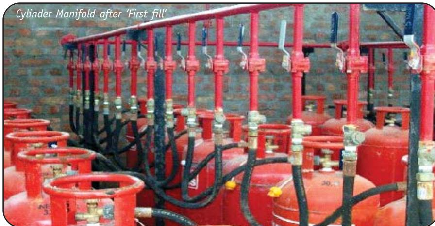
*Cylinder Manifold after ‘First fill’*
